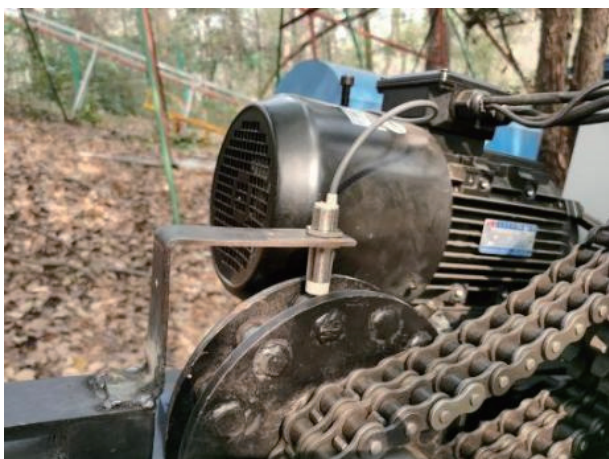
Figure 9 Proximity switch installation
