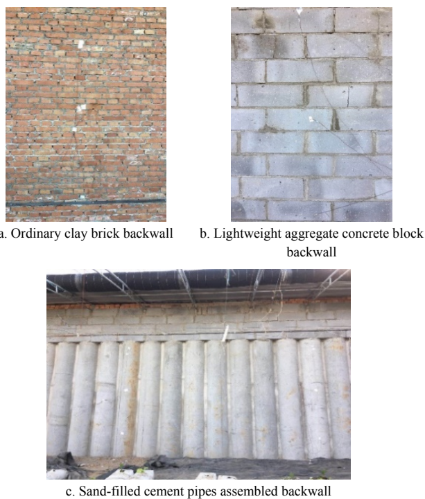
Figure 2 The backwalls tested in this study
