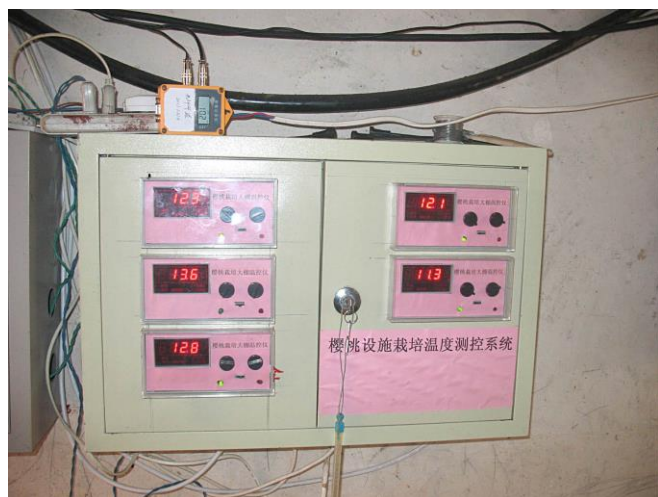
Figure 5 Working state of the temperature measurement and control system for sweet cherry facility cultivating
