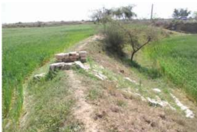
Figure A4 Loose stone structure in the field
