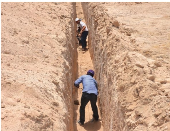
Figure 2 Preparation of the slope for the pipes
